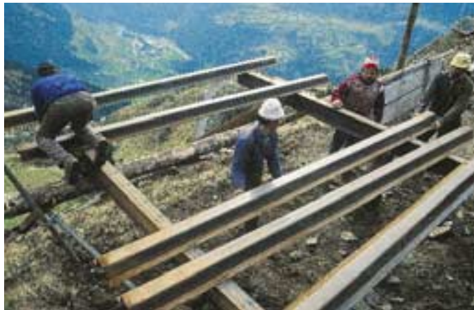
Installation of an avalanche protection barrier above Airolo (TI).
